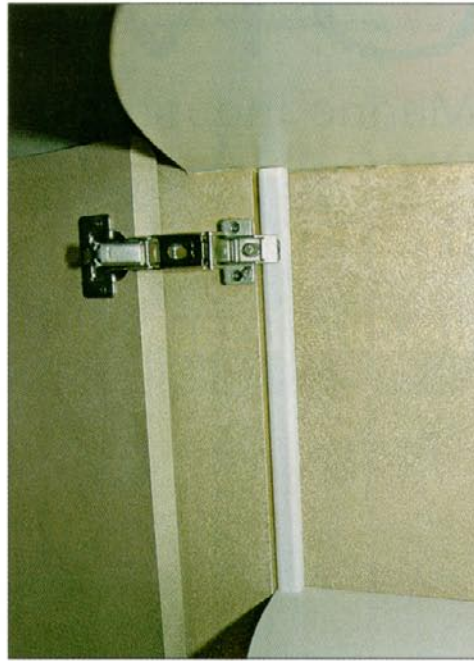
Far left —Unexpected's engineroom is accessed through a solid door front and a cored horizontal hatch. Left —Drilling additional shelf support-pin holes in the installed panels proved difficult, so Evans added support posts to the cabinet sidewalls underneath the shelves.
